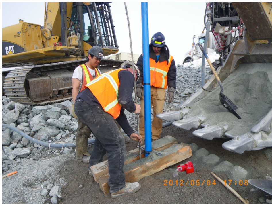
Photo 2: Installation of ND-IN-070-2. A length of rebar was used to ensure the sand did not bridge down the borehole.
