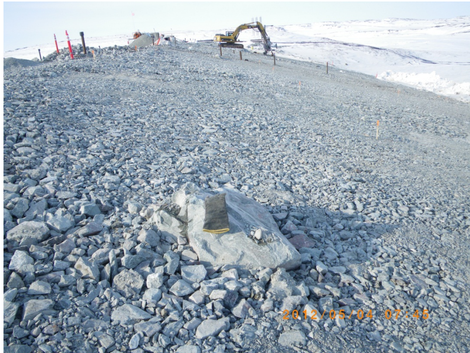
Photo 1: Large ROQ boulder installed as a Surface Settlement Point. The Survey pin to be installed.
