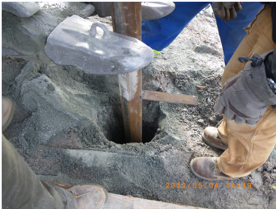
Photo 3: The foot welded to the side of the protective housing to ensure it is installed at the correct elevations.
