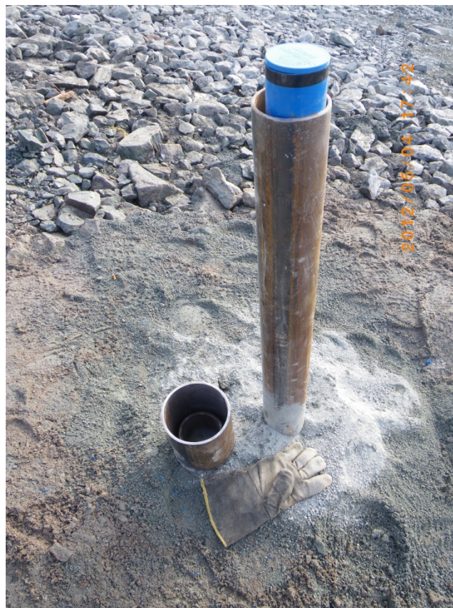
Photo 3: The completed stick-up of ND-IN-070-2.
